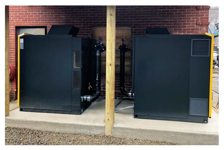
DBS screw blowers with variable frequency drives helped Chapmanville Water Department lower its energy expenses while also upgrading its failing blowers.
