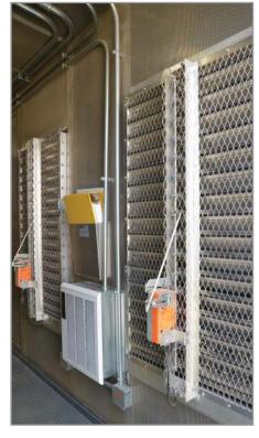
Thermostatically controlled louvers and enclosure heaters
